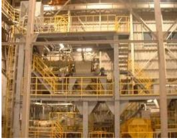
Automobile catalyst sampling facility
