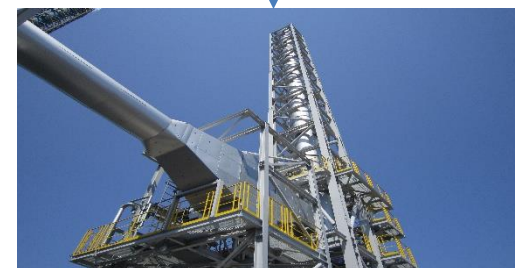
New incinerator in Yokohama
