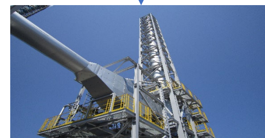
New incinerator in Yokohama
