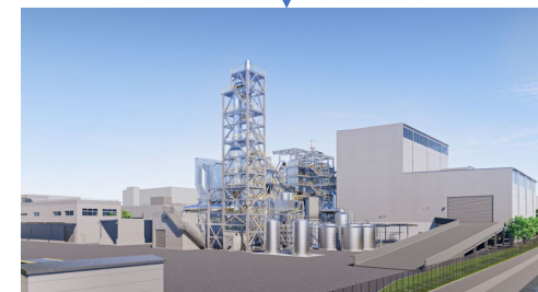
New incinerator in Yokohama
