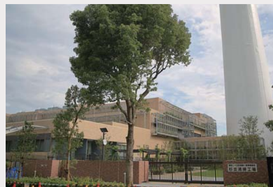
Suginami Incineration Plant
