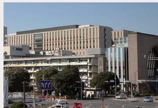
Keio University Hospital New Hospital Wing (Building 1)
