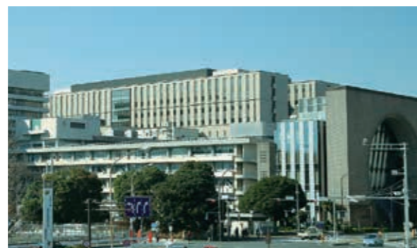
Project example: Keio University Hospital New Hospital Wing (Building 1)
