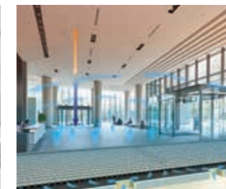
Floor radiant air conditioning systems
